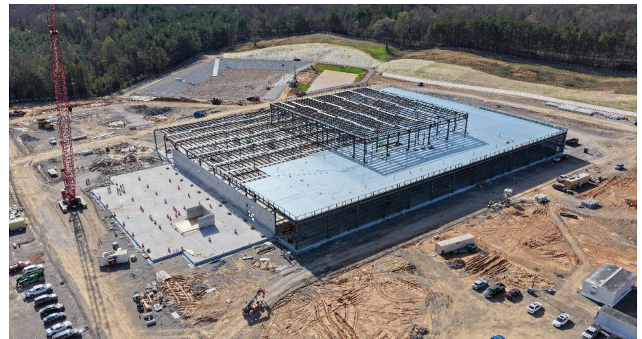
Current TX-1 Vertical Construction Progress
