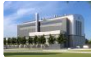
Hermes 2 (Phase 2): Large-scale Precast Production (4,000 pieces)
