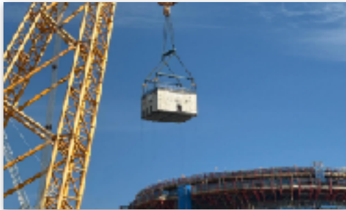
Above: Modularisation now includes whole pre-cast rooms,
