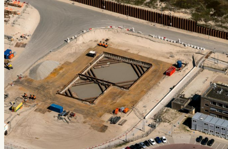
Aerial overview of the SCS building pit
