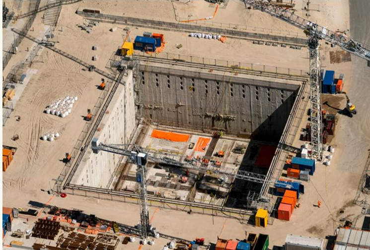
Aerial overview of concrete pouring -3 floor Nuclear Island
